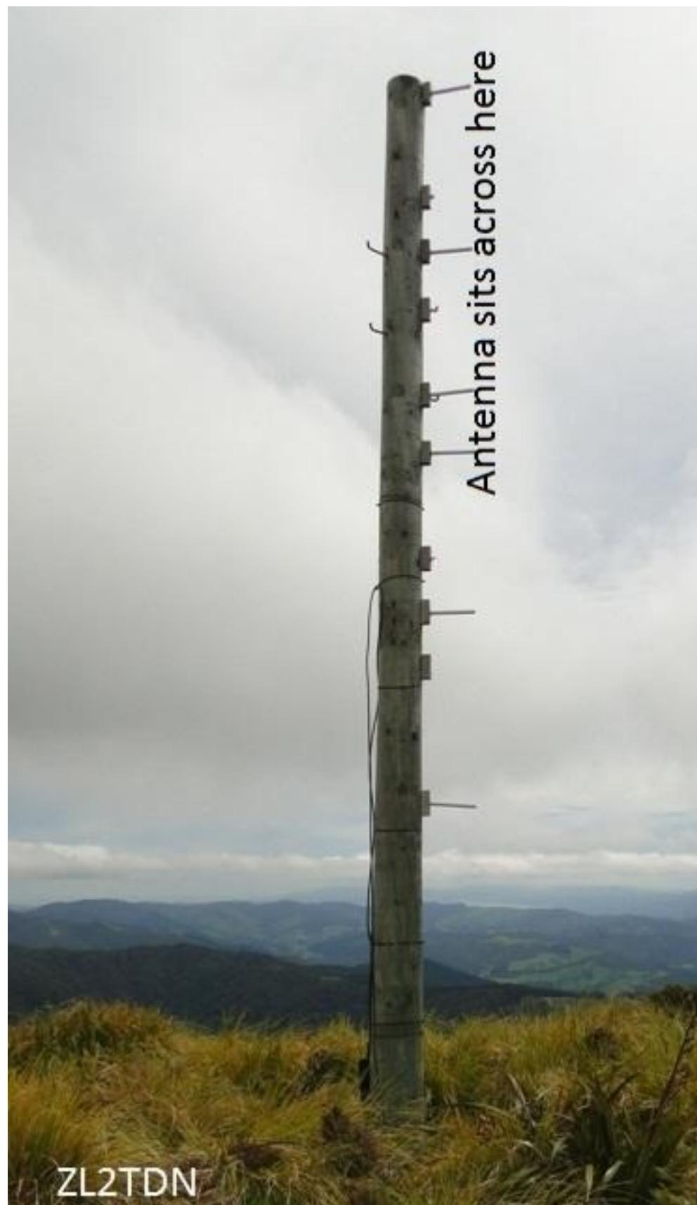
The match isn't quite as good as expected forward power 74 watts reflected 4 watts; a choke was attempted making a loop of 4 or five turns of coax about 120mm diameter cable tied together. This needs further work but the results have been most satisfying so far. It will be interesting to see if the summer temperatures cause any detuning. The radiation angle should be a lot lower than the previous one and the capture area will be increased.
