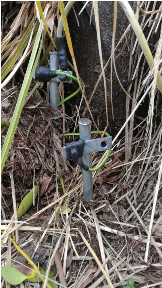
Picture-4: Earth stakes in parallel 29 th September 2019.
